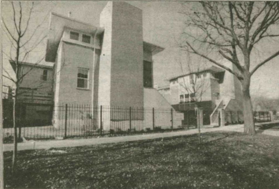
The Plaisance Place located on 61st and Greenwood, is the first new construction in the Woodlawn community setting the stage for more new construction to follow attracting more middle income families.
