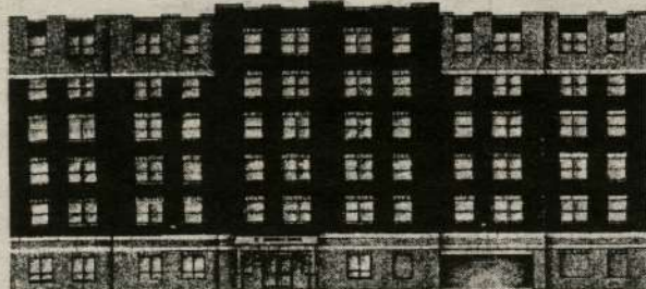
St. Edmund's Tower, a senior housing complex to be located at 6141 S. Michigan Ave.
